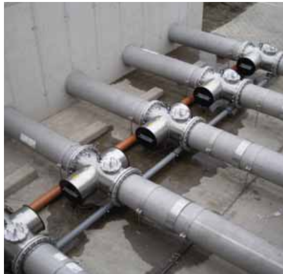
Szeged, Hungary 5 x bersonInLine 1500 + WW 5000 m 3 /h wastewater disinfection to meet EU-bathing water directive
