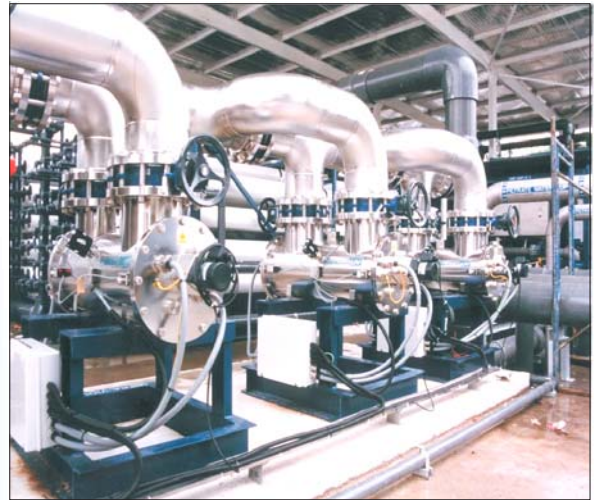
Bedok Effluent Re-use Plant, Singapore
